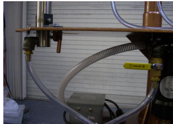
8. Vacuum is supplied through individual valve.
